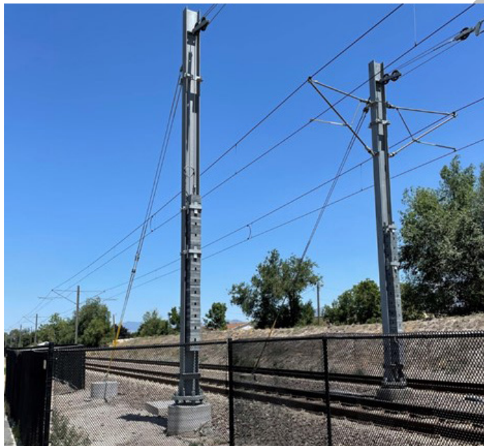
UTA SOGR project - New BWA in existing ROW
