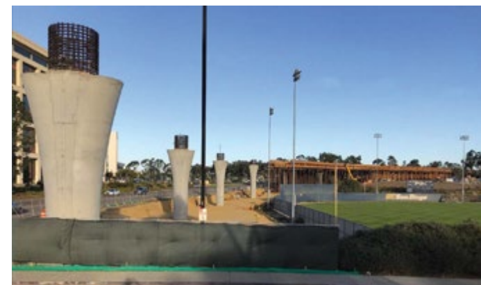
Breaking Ground: Mid-Coast Trolley Extension
