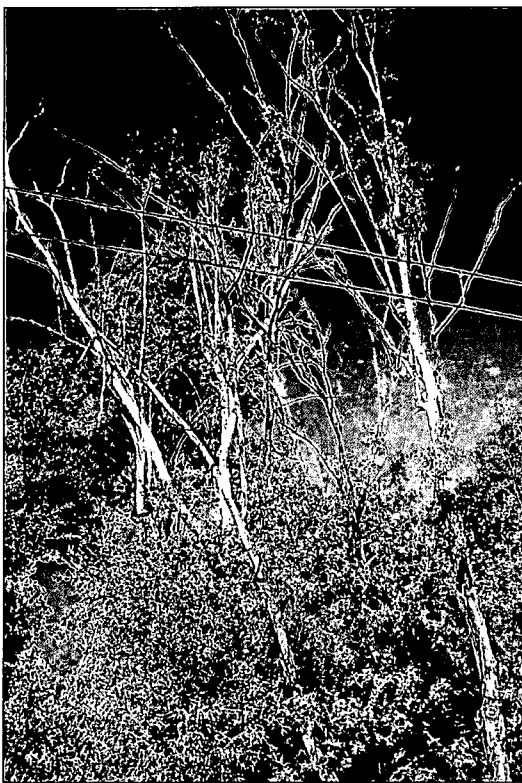
Figure 32: Overgrown Trees Interfere with Catenary Wires
