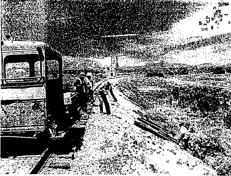
Cleaning ROW of rotten ties @ MP 66.8 looking east
