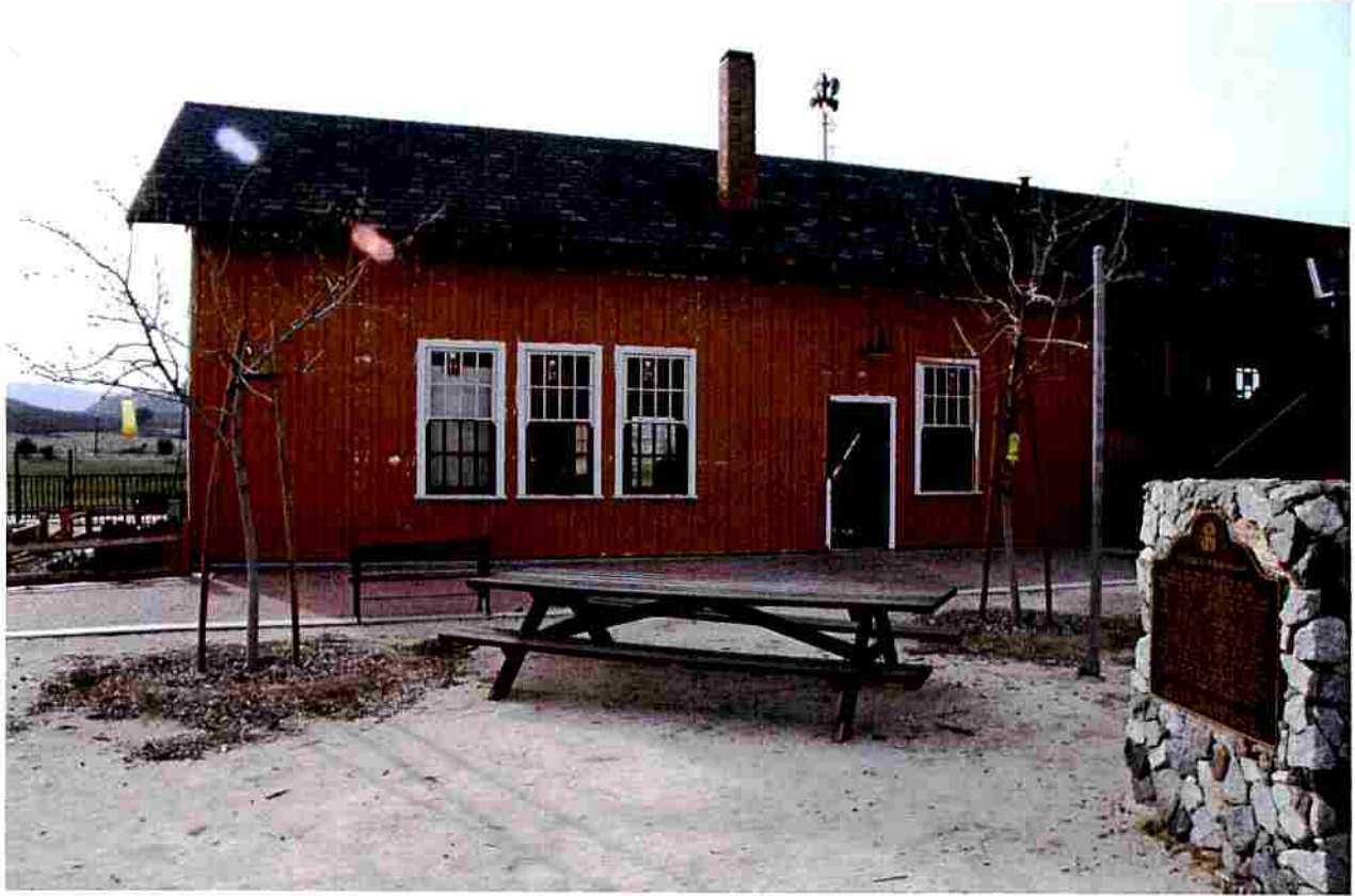
South side Campo Depot Exterior restoration nearly complete
