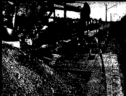
Platform Improvements In Progress – Trenching for Conduits and Shelter Foundations
