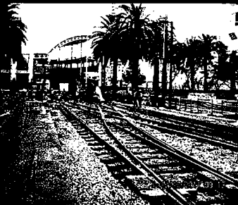
Installation of the Double Crossover
