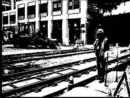
Trackwork on C Street and India Street
