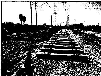
Concrete Tie Replacement
