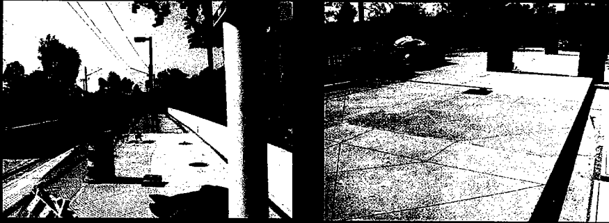
Platform Improvements In Progress
