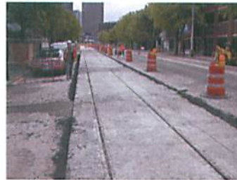
Paved Track Nearing Completion
