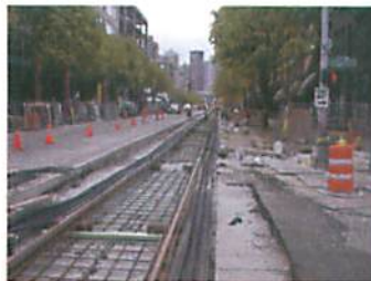
Guideway and Track Construction
