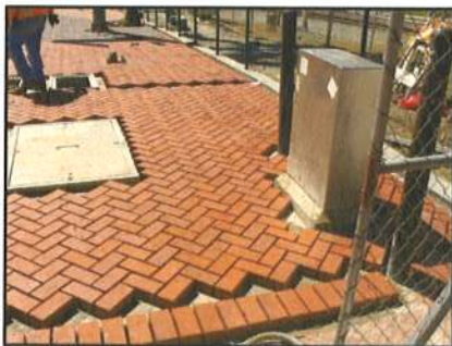
South Platform - Brick Pavers in Progress
