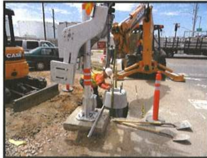
Installation of Precast Signal Pedestal
