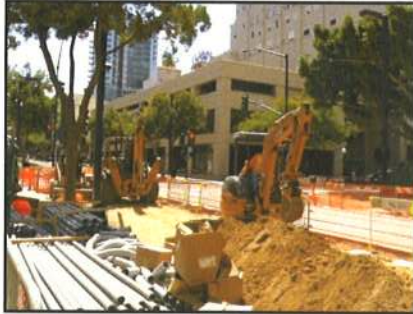
North Platform Demolition and Conduit Trenching
