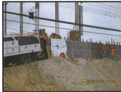
Retaining Wall for Signal Cabinets
