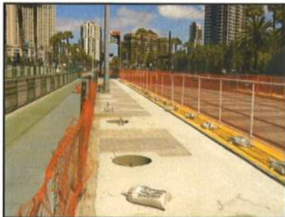
South and North Shelter Foundations and Platforms - Ready for Granite Pavers
