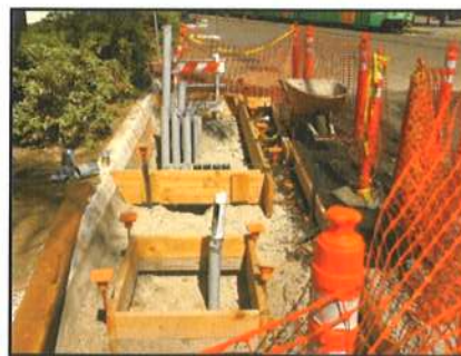
Duct Bank to Building A in Progress
