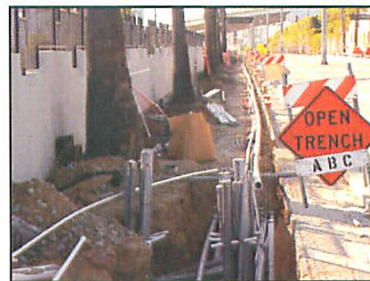
Conduit Installation – Both Platforms
