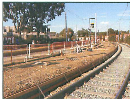
West Bound Platform Open for Boarding - Conduit Installed and Forming East Bound Platform for Improvements
