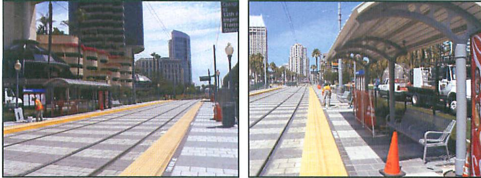
Platform Paving Completed and Shelters Installed - Opened for Low Floor Boarding
