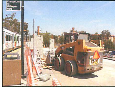
Demolition of Shelter and Platform in Progress
