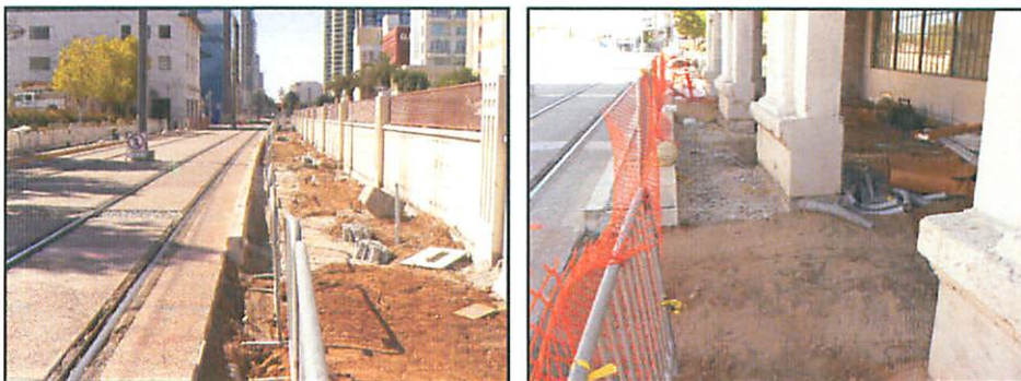
Station Construction in Progress - Demolition and Placement of Conduits Completed
