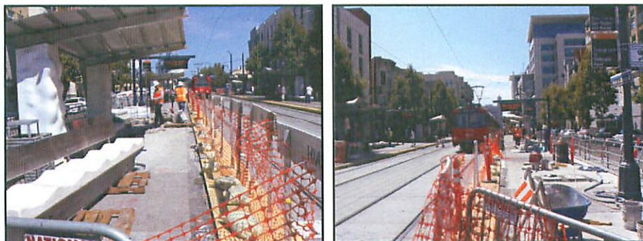
East Bound Platform - Paver Installation in Progress and Track Side Boarding - West Bound Platform
