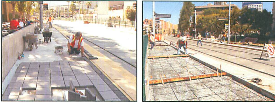
Station Closed During Construction - Placement of Pavers in Progress
