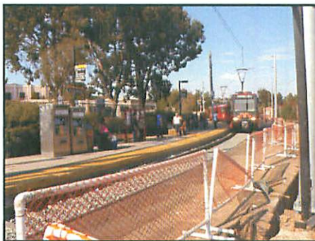
West Bound Platform Open for Boarding - Conduit Installed and Forming East Bound Platform for Improvements
