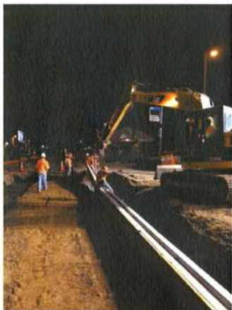
Construction of Turndown Slab (For New 8 th Street Platform)
