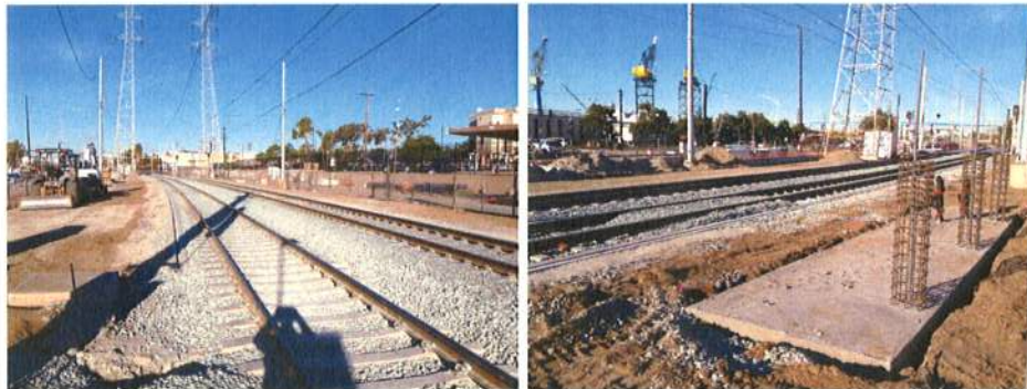
Trackwork Complete in both WB (NB) & EB (SB) Directions Site Prep for Platform Pours & Rebar Cages for Shelter Column Pedestals
