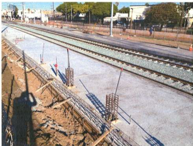
Completed Platform Slabs with Rebar Cages for Shelter Column Pedestals
