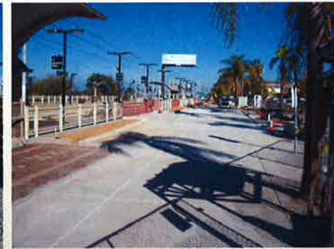
Flatwork Behind Station Remaining
