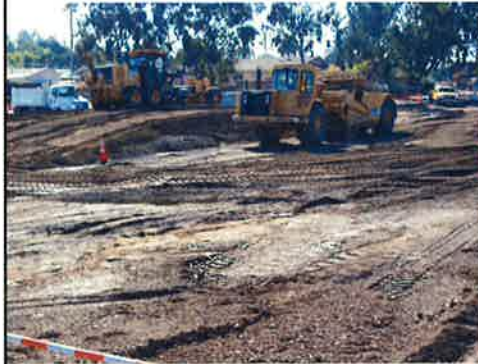
Demolition & Grading in Parking Area
