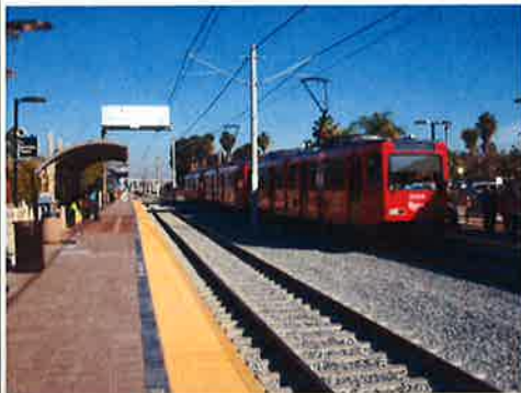
Platforms & Trackwork Complete
