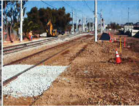
Beginning Construction of Temporary Platform
