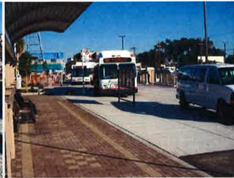
Bus Transit Center Complete.... Finishing Parking Lot
