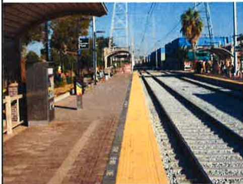
Minor Work at North End of Each Platform Remaining
