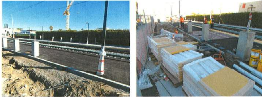
Installation of Platform Pavers & DWP's
