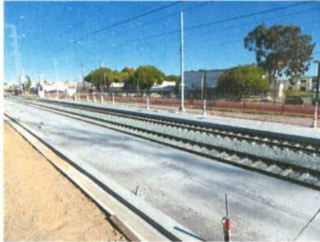
Platforms Ready for Installation of Shelters, Pavers & DWP's
