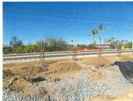
Platform Grading & Shelter Pedestals
