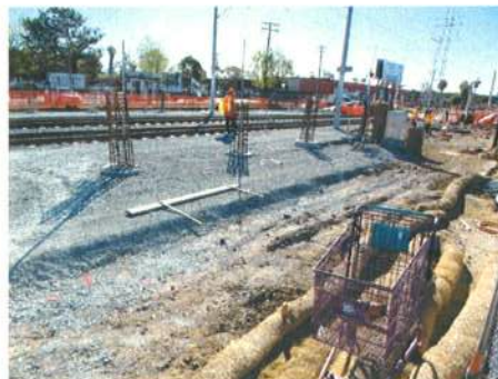
Platform Grading and Shelter Pedestals
