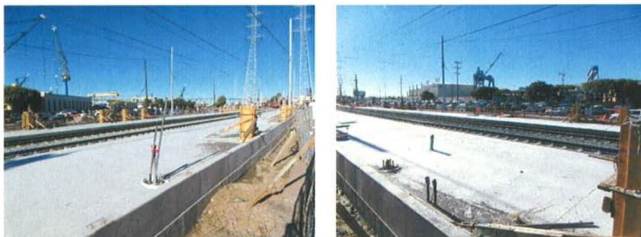
Platforms Ready for Installation of Shelters, Platform Pavers & DWP's
