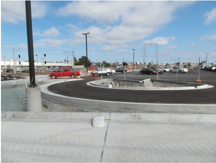
Curb & Gutter and Asphalt Pavement in Parking Lot and Bus Turnaround
