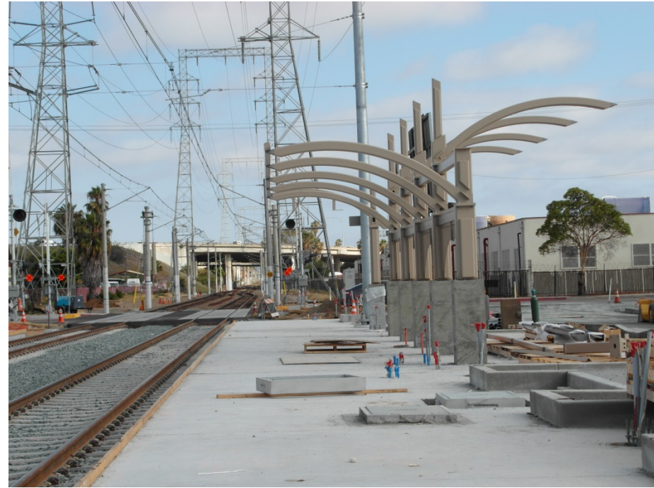
Platform Ready for Pavers and First “Double Gull Wing” Shelter Being Installed
