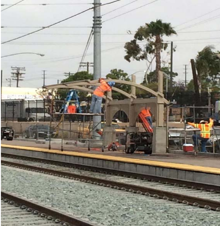
Installing Shelters and Pavers
