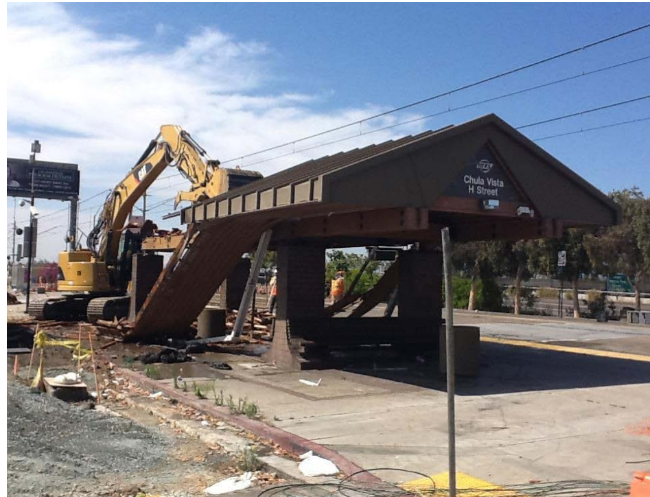
Demolition of Existing Platform & Shelter
