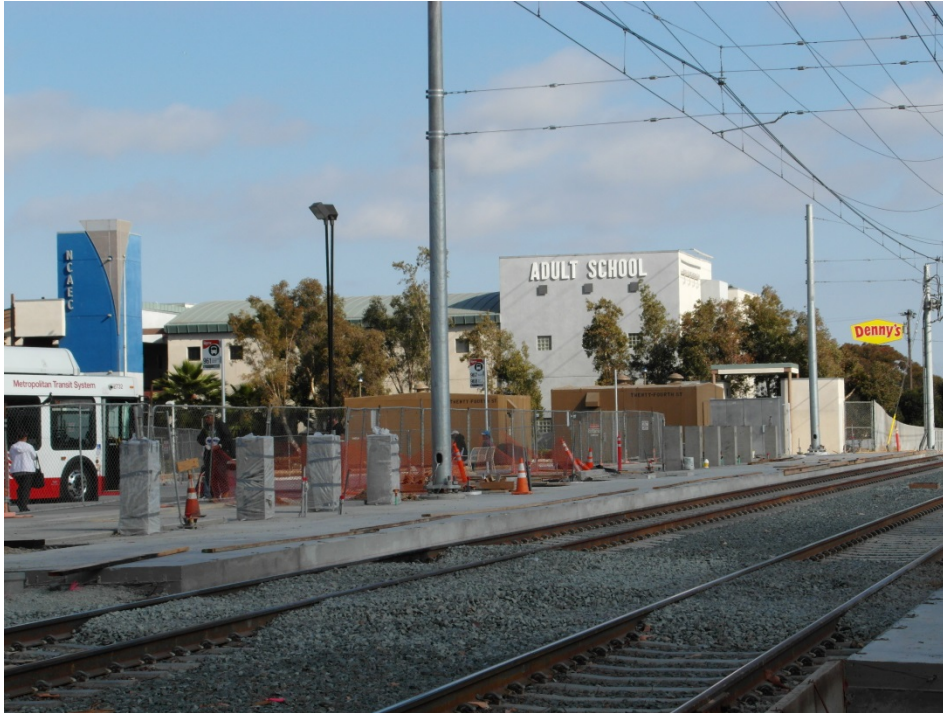
Platforms Ready for Pavers and Column Pedestals ready for shelters
