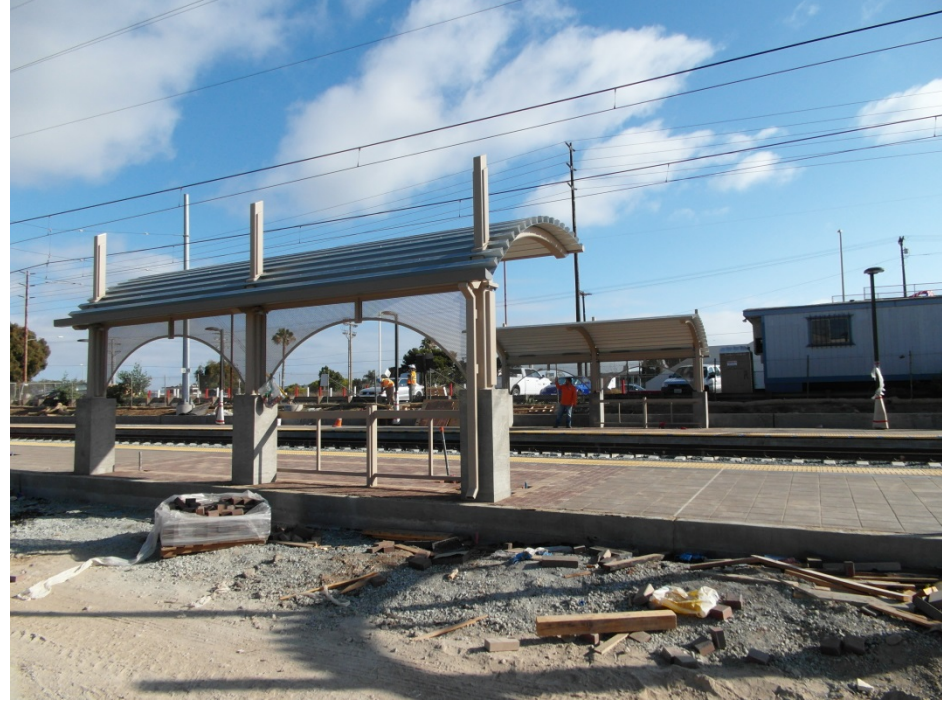
Shelters and Platform Pavers Nearing Completion
