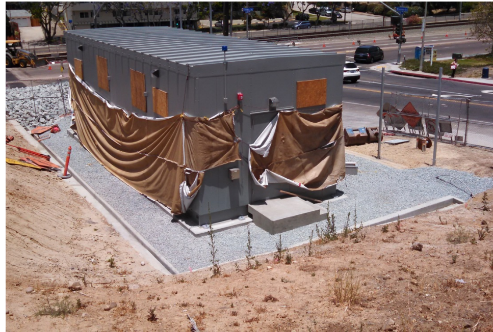
TPSS Installed and Ready to be Energized @ 66 th & Imperial (Woodman site)
