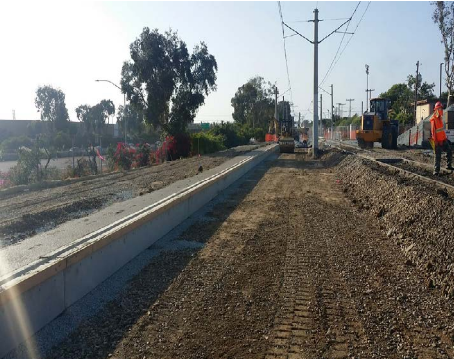
Excavation & Installation of Turndown Slab for SB Trackway Replacement
