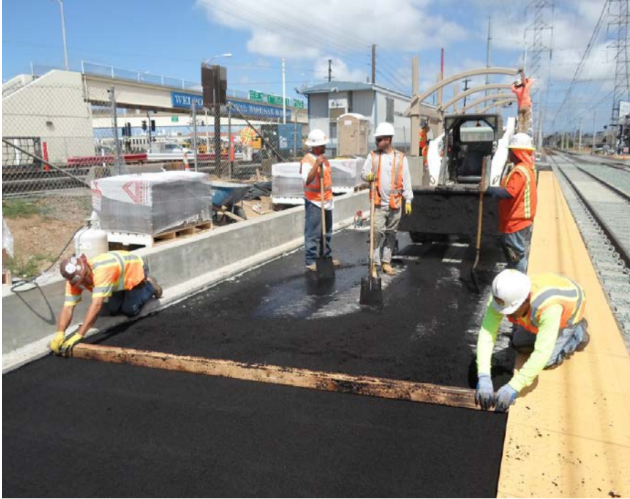
Installing Shelters and Laying Bituminous Bed for Pavers
