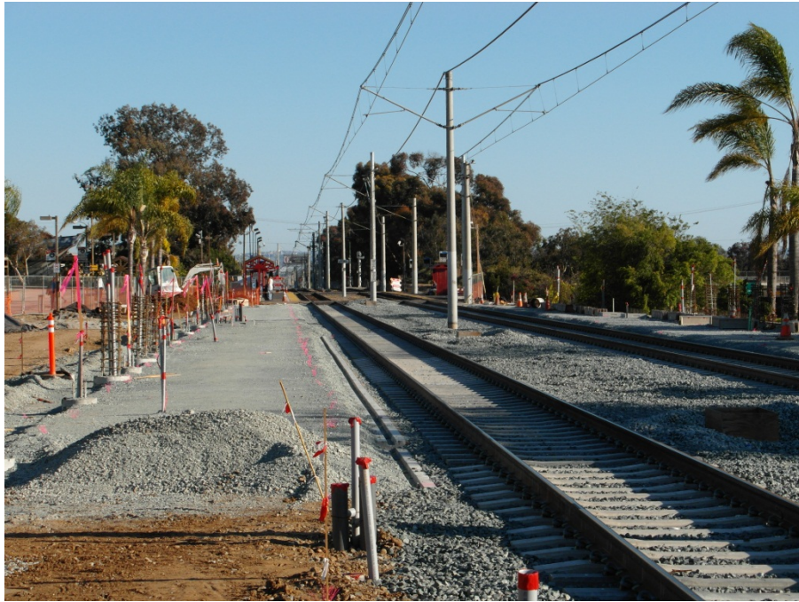
Forming Eastward (SB) Platform and Shelter Pedestals
