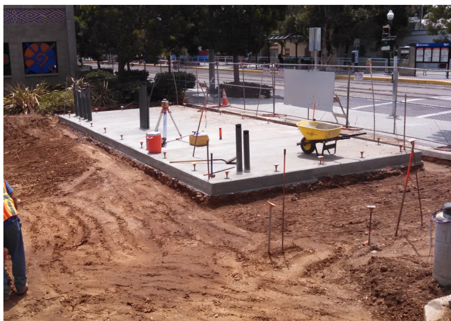
Ground Grid Installed & Pad Ready for TPSS Installation @ 25 th & Commercial (Police Station site)
