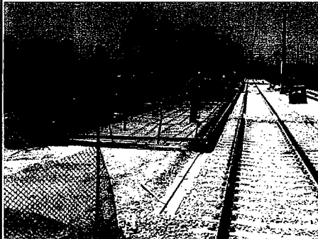
Forming & Pouring Concrete Platforms
