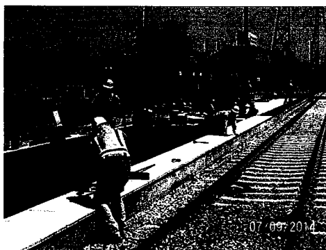
Installing DWP's and Preparing Platforms for Pavers
