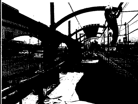
Installing Shelters & "Touching-up" Welds
