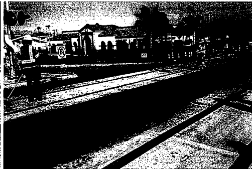
Newly Replaced H Street Grade Xing (Over 2 Weekends of "Single-Tracking")
