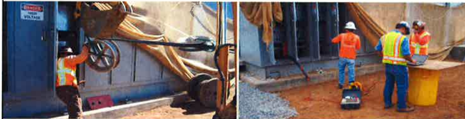
Pulling & Testing Feeder Cable for TPSS @ Main Street
