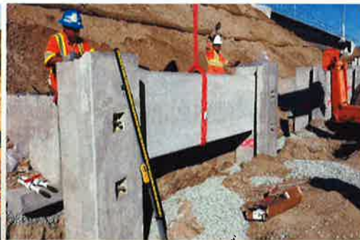
Constructing Precast Concrete Counterfort Retaining Wall for Extending Siding Track @ Main St. in Chula Vista
