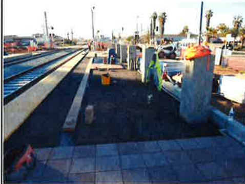
Installing Platform Pavers on EB Platform
