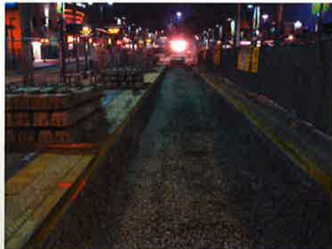
Excavated Trackway down to subballast and replaced with new Ballast, Concrete Ties, Rail and Concrete Finish so Top/Rail could be lowered to accommodate New Low Floor LRV's
