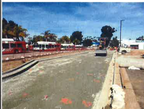
Fine-grading Base in Bus Transitway
