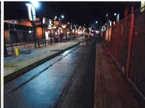
Excavated Trackway down to subballast and replaced with new Ballast, Concrete Ties, Rail and Concrete Finish so Top/Rail could be lowered to accommodate New Low Floor LRV's
