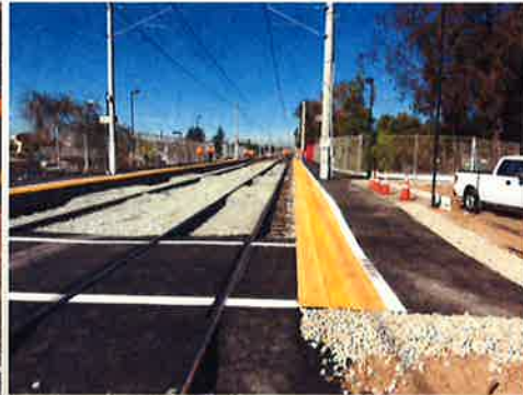
Completed Temporary 8" Platforms ready for New Low Floor Service
