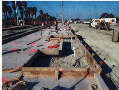
Completing Planter Curb on WB Platform Prior to Setting Pavers
