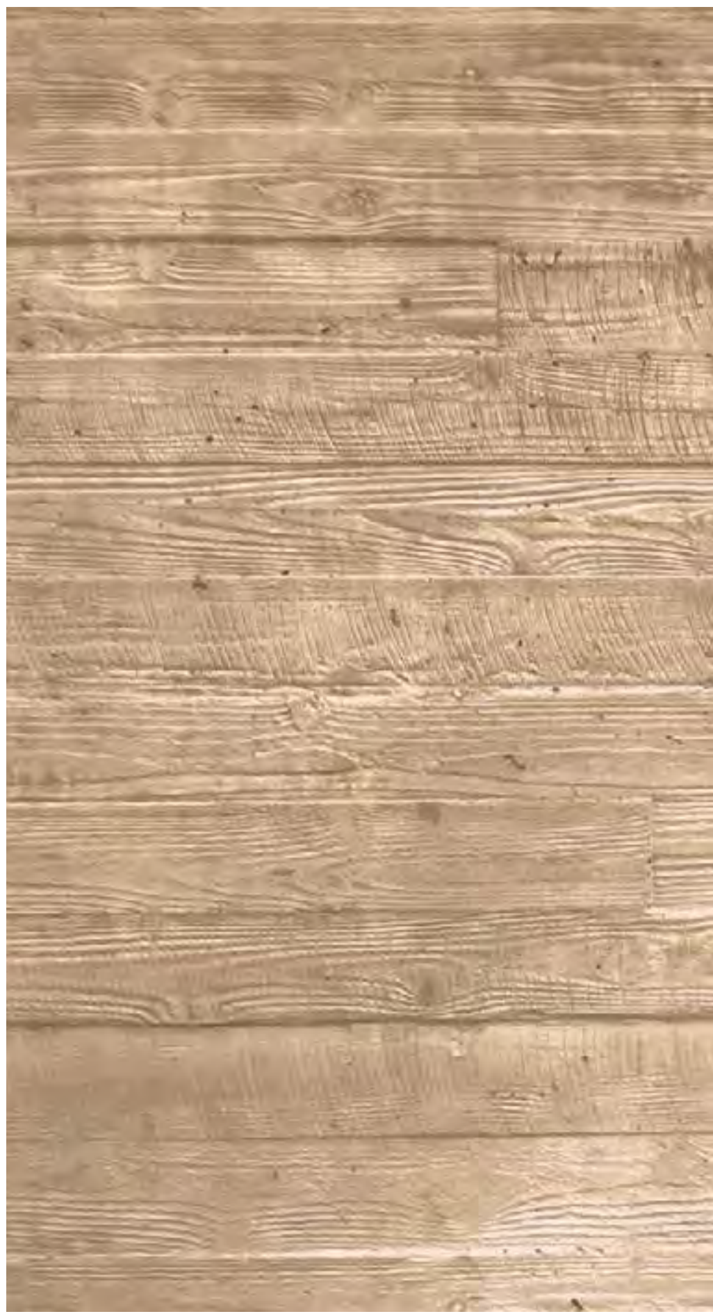
BOARD FORM CONCRETE WITH INTERGRAL COLOR BUFF
