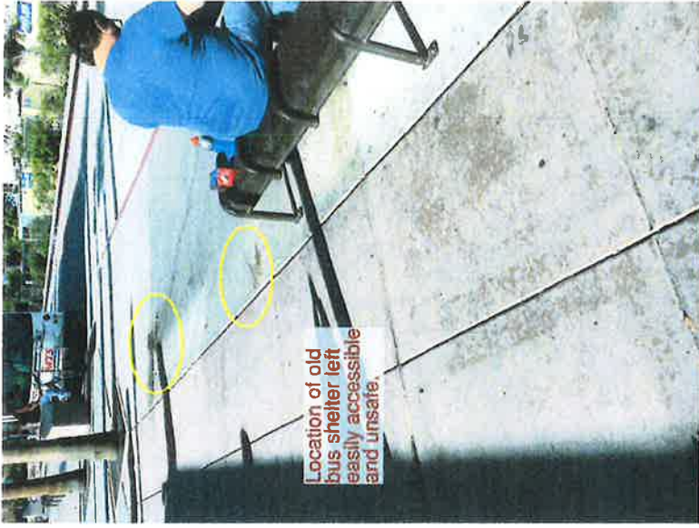
Live conductors were simply taped and stuffed into conduit at ground level and left accessible by the public
