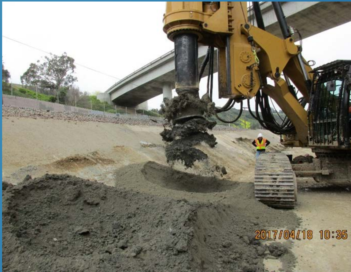
Drilling 30 inch CIDH Piles in Rose Creek Channel in Reach 9
