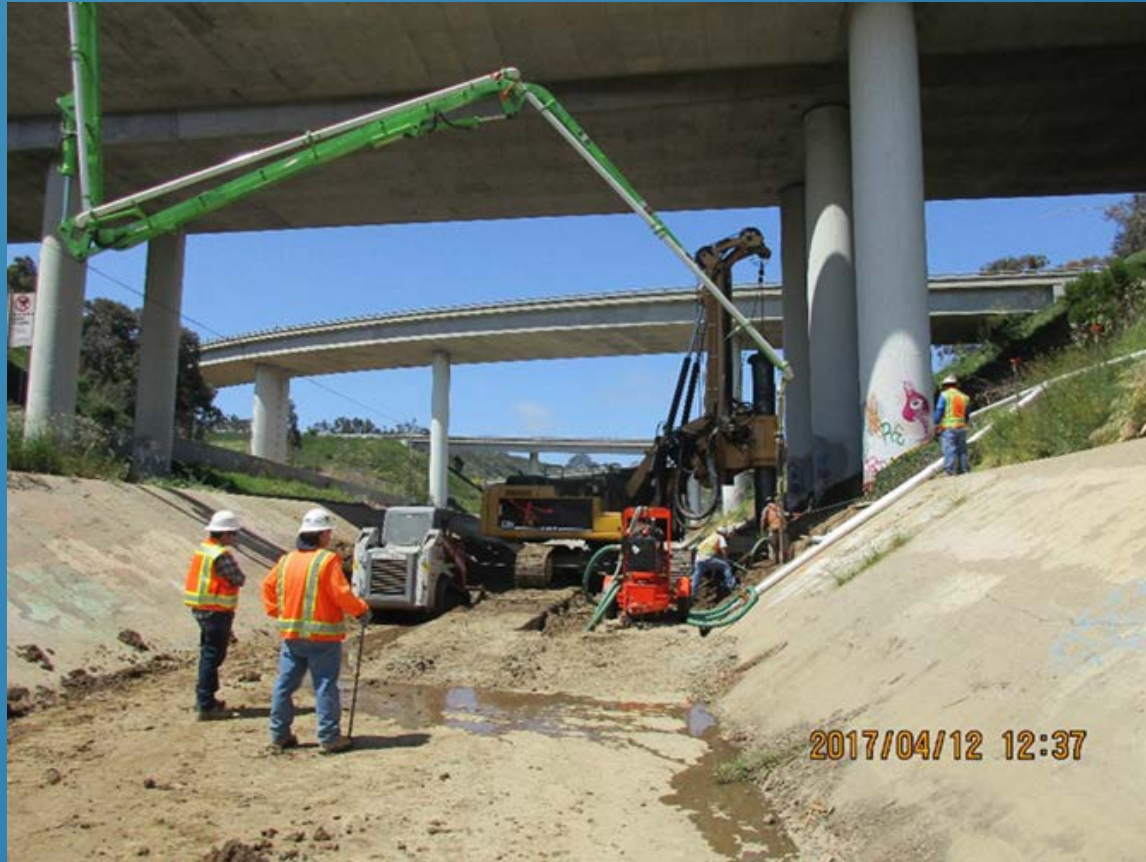
Drilling for 30 inch CIDH Piles in Rose Creek Channel in Reach 9
