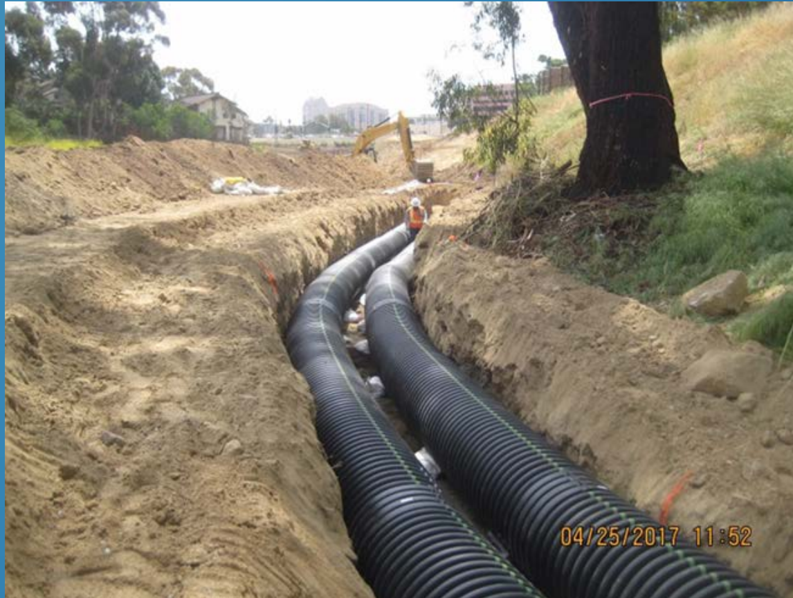
Temporary Drainage Diversion within Pepper Canyon to facilitate Bent Construction
