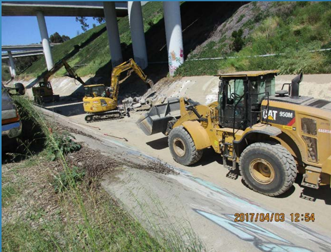
Wall Concrete Slab Removal at Rose Creek U Channel in Reach 9
