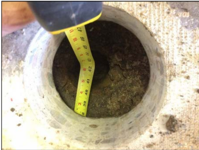
TAPE MEASURE DEMONSTRATING AIR GAP BELOW CORING C6
