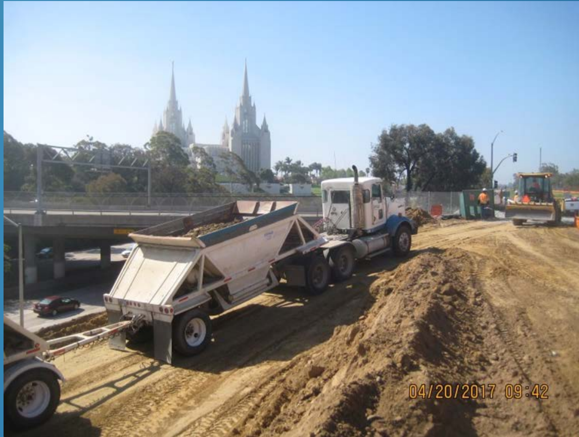
Exporting Material from Whole Foods Slope to SR-11 to establish Nobel Viaduct Bent Access
