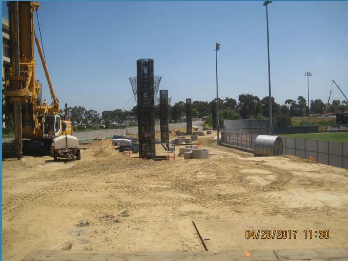
Bent Columns Reinforcement Cages being installed behind UCSD's Trident Field
