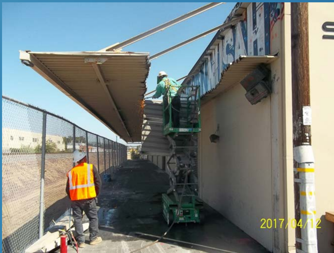
Removing Overhead Canopy at Loading Dock in Reach 4 by Anna Avenue
