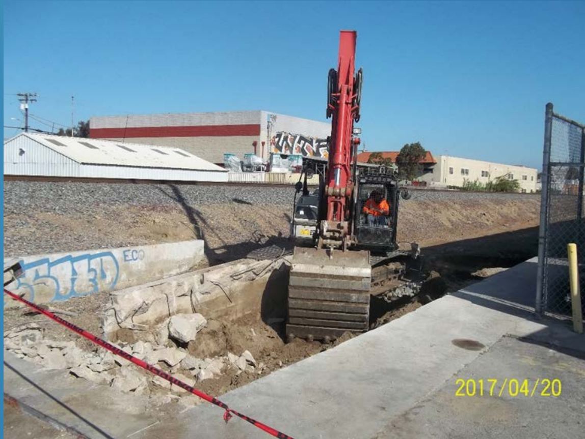
Removing Retaining Wall at Loading Dock in Reach 4 at Anna Avenue
