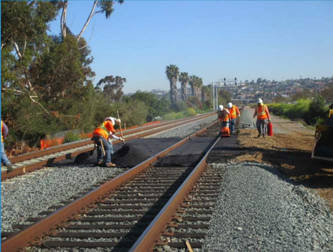
Paving Temporary Crossing at Sta. 282_30 in Reach 5
