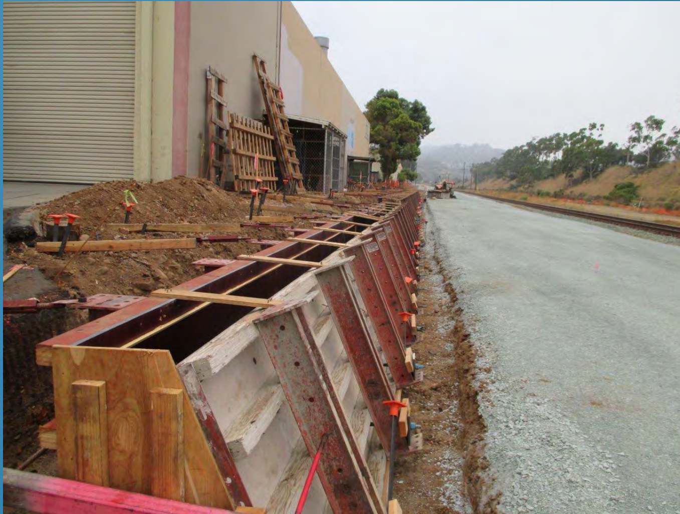
Rose Canyon Project Construction – Railroad Base Preparation & Gravity Wall
