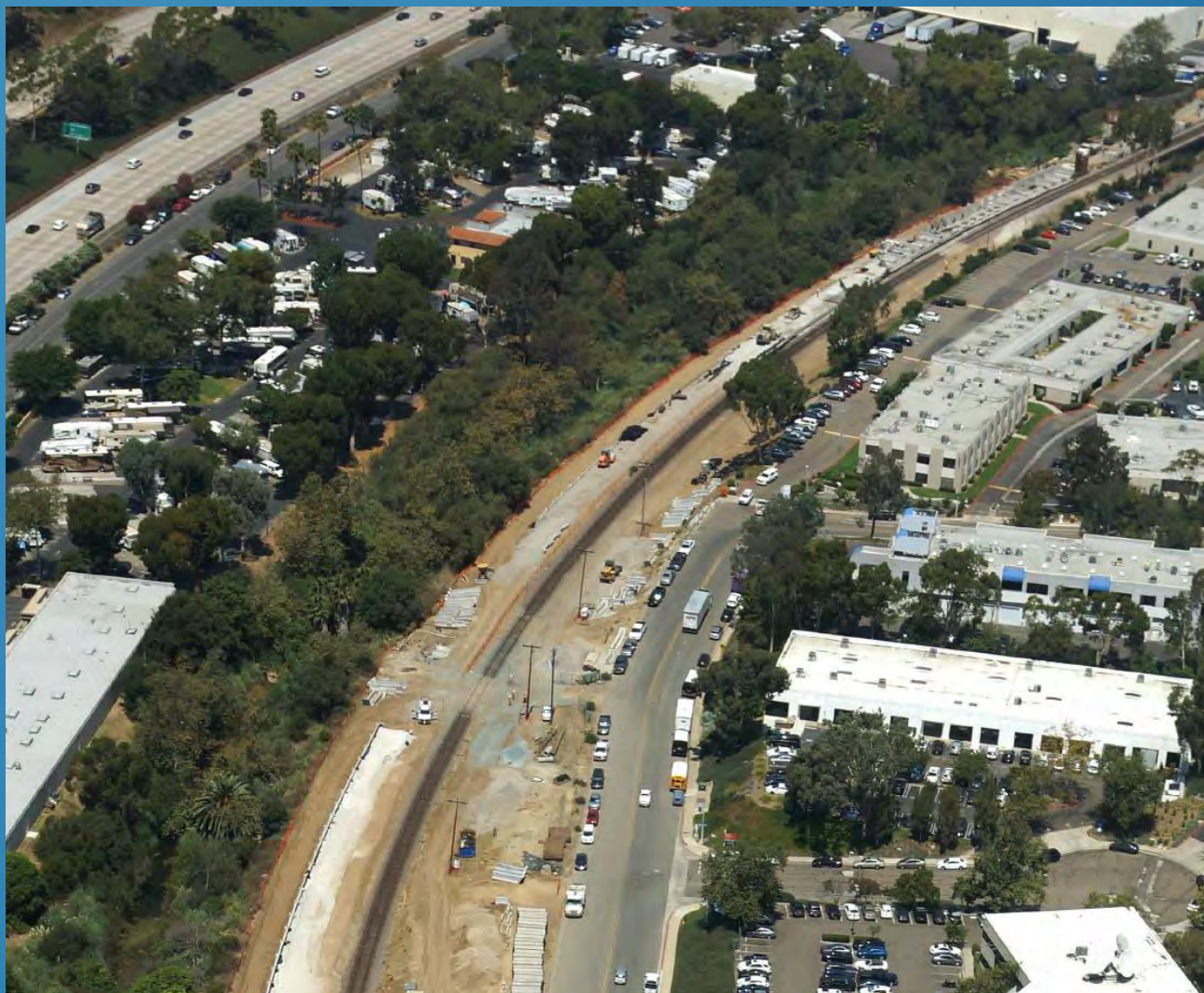
Rose Canyon Project Construction – Clearing and Counterfort Walls
