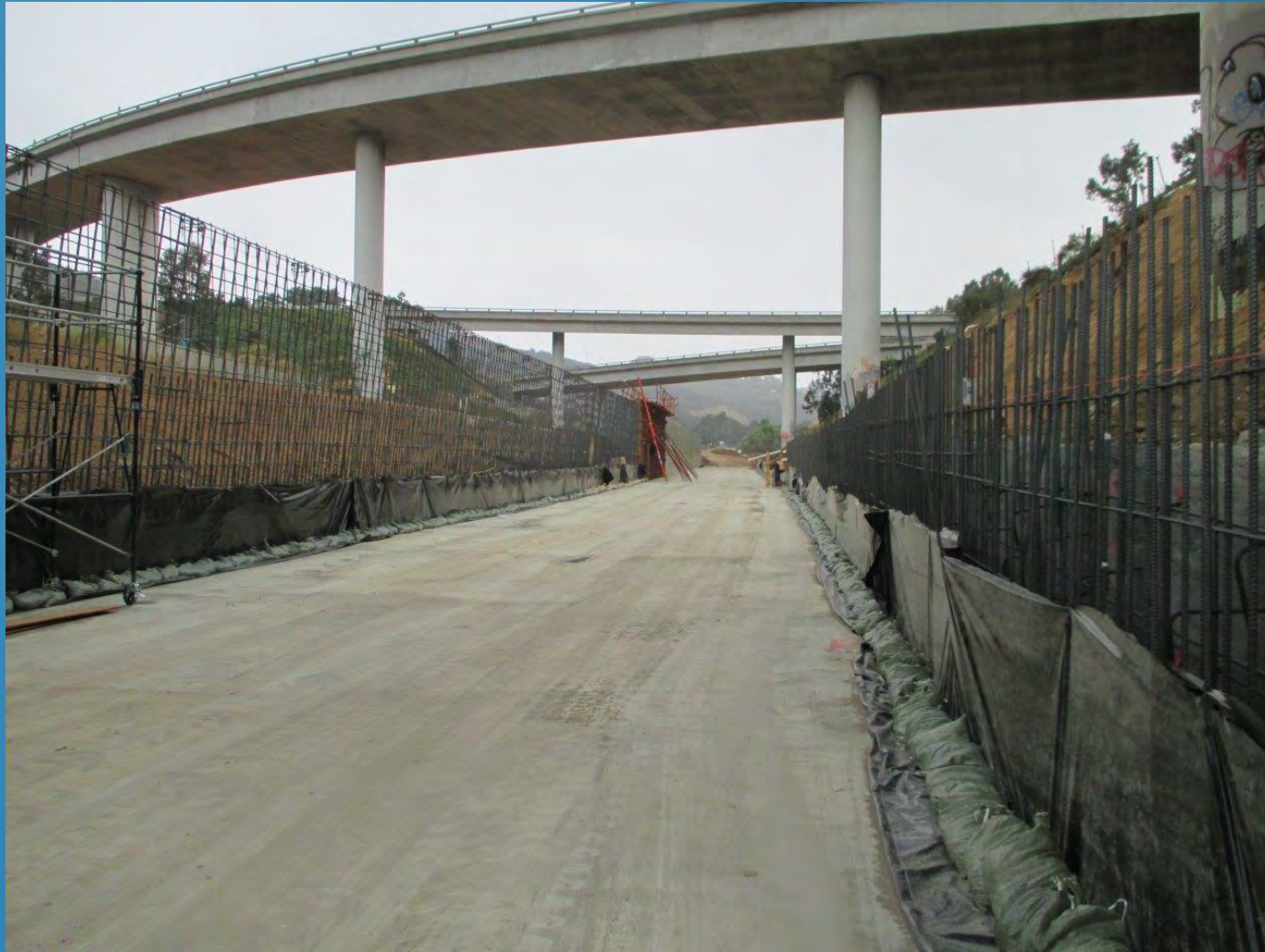
U-Channel Construction under SR-52
