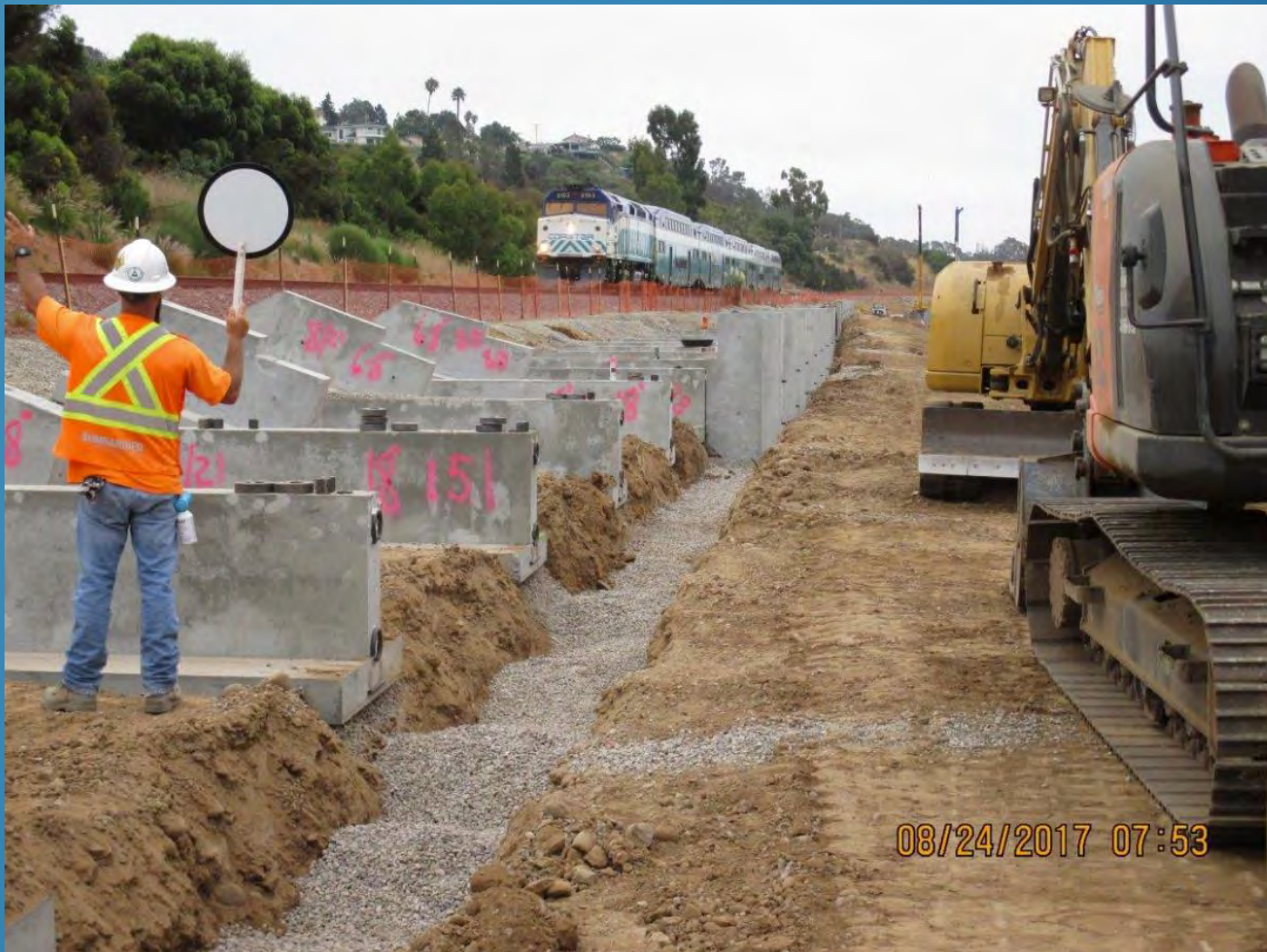
Rose Canyon Project Construction – Clearing and Counterfort Walls
