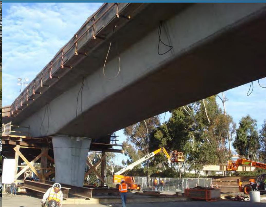
UC San Diego Viaduct – Removing Falsework
