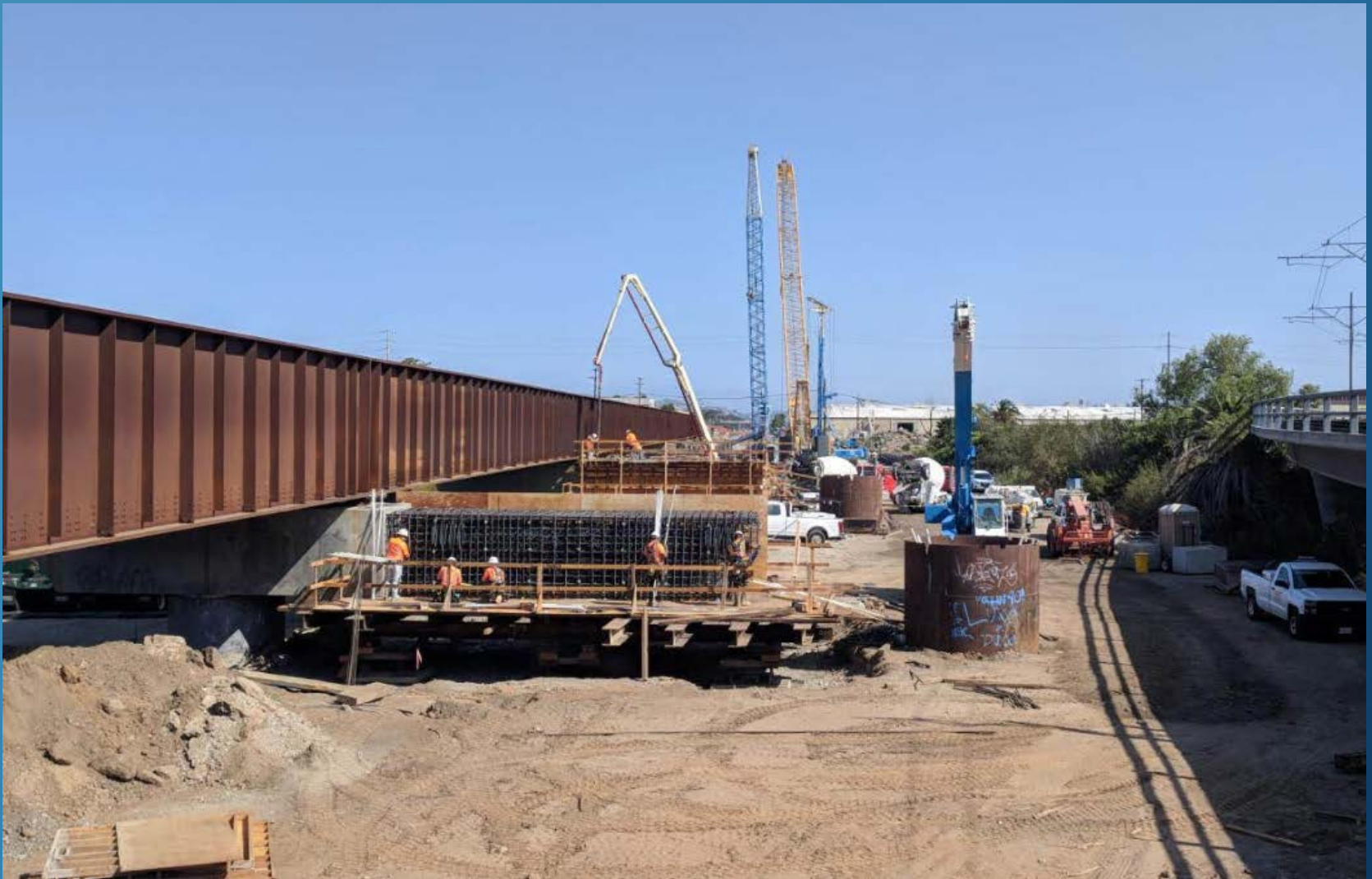
LOSSAN Bent Cap & LRT Column Construction
