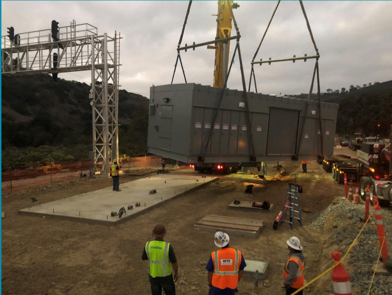
First TPSS Installed on Project
