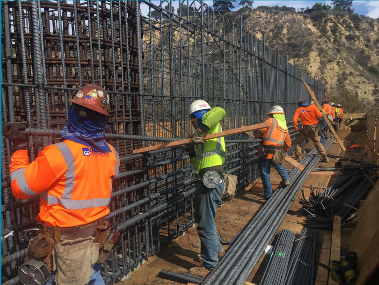
LRT Flyover by Karl Strauss – Rebar Cage Construction
