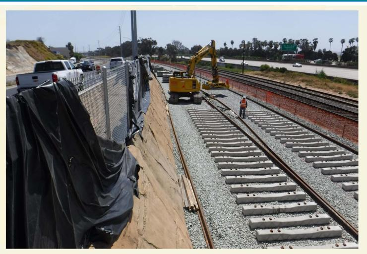
Setting Concrete Ties and Continually Welded Rail
