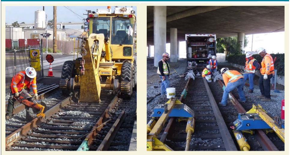
Installing Insulated Joints during AWW in Reach 1
