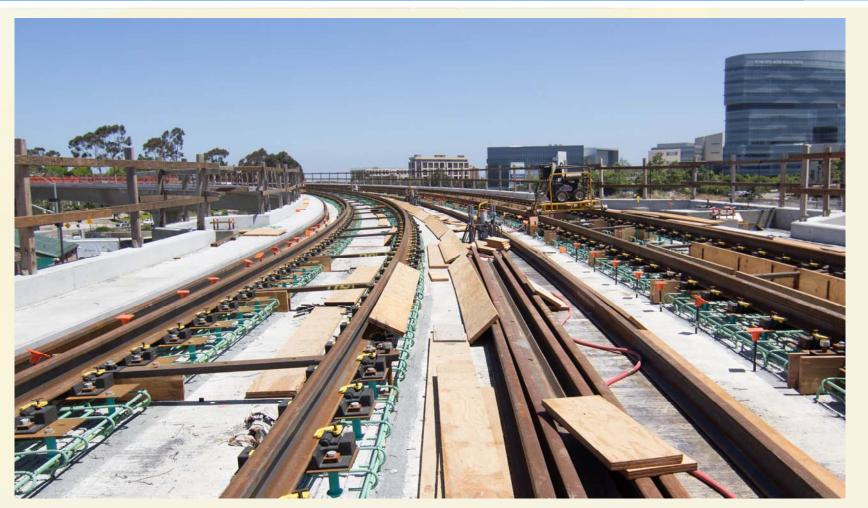
Direct Fixation Trackwork of UCSD Viaduct
