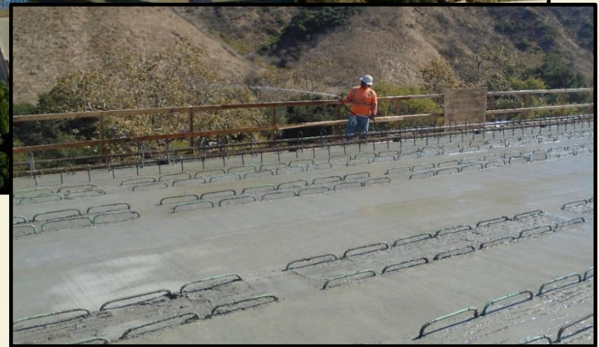
Curing Rose Creek LRT Flyover Bridge
