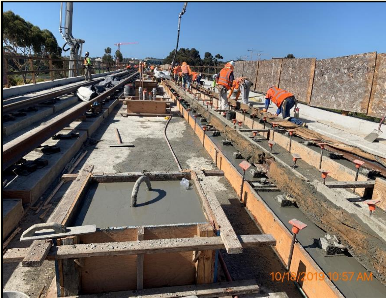
Placing OCS Foundations and Plinth Concrete – UC San Diego Viaduct
