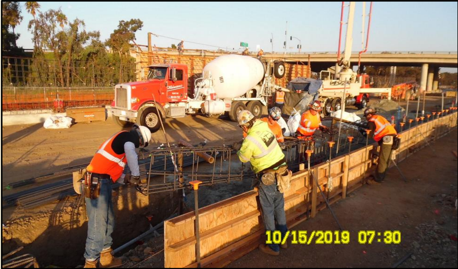
Tecolote Station Northbound Fence Foundation
