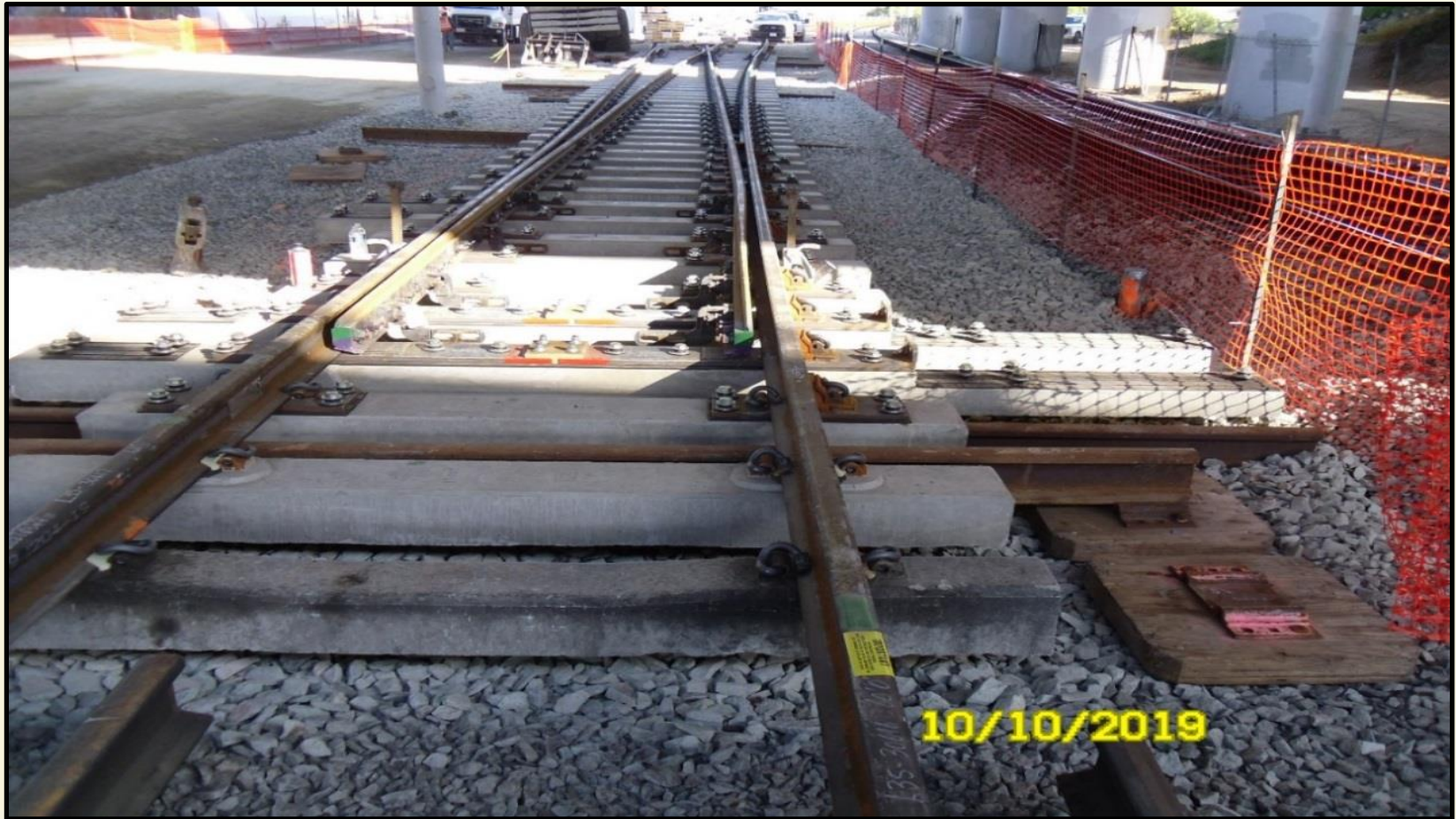
Green Line Tie In Switch Construction
