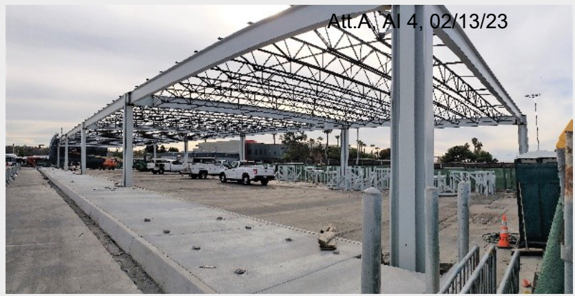
Overhead Charging Frame in Construction at South Bay Maintenance Facility
