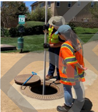
Inspection of a Hydrodynamic Separator Unit
