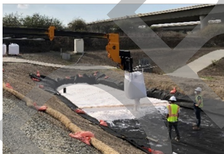
WSP provided on-site construction oversight of the Austin Sand Filter retrofit to ensure that the treatment BMP was installed per plan.
