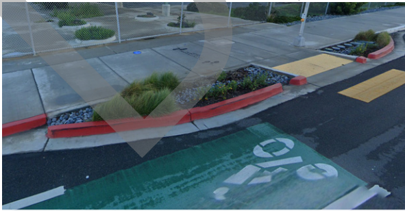
Bend out roadway treatment incorporating a green gutter
