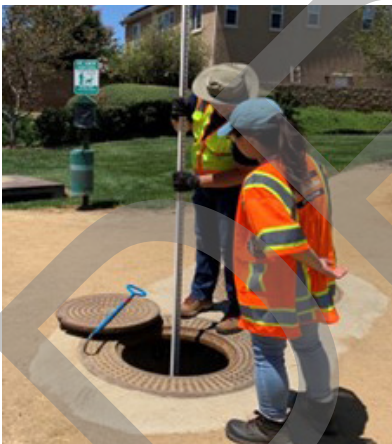
Inspection of a Hydrodynamic Separator Unit
