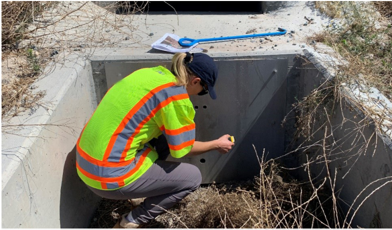
Inspection of a Bioretention Basin with Hydromodification Flow Control Orifice
