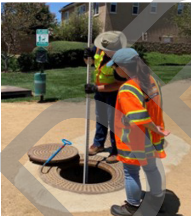
Inspection of a Hydrodynamic Separator Unit
