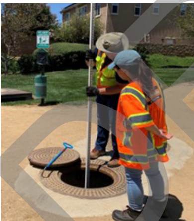
Inspection of a Hydrodynamic Separator Unit
