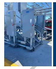
Untimely conduction analysis of OPD coordination study resulted in added electrical equipment (current limiting devices) which resulted in added contract change order costs and added workdays to the contract schedule
