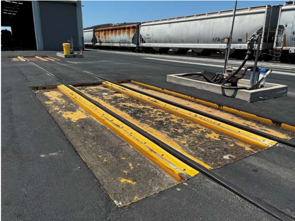
Pump island and secondary containment for T002
