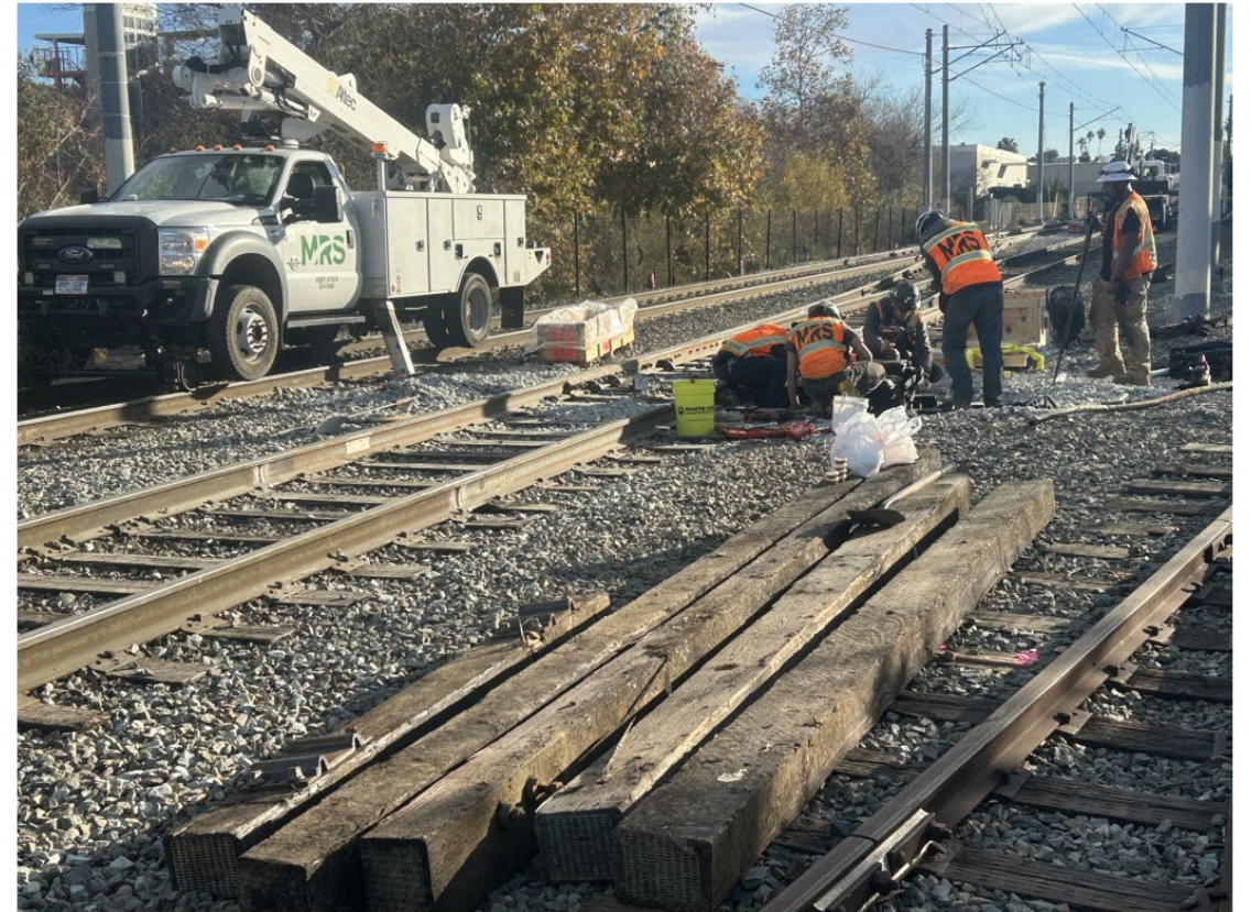
Sunday, January 18, 2026, 3:30AM: Work continues at Switches E315A/B wiring switch mechanisms.
