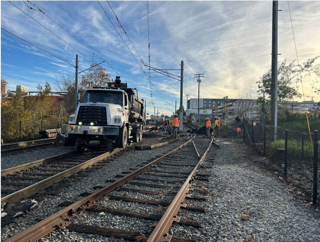
Saturday, January 17, 2026, 8:03AM: Switches E315A and E315B being removed east of Euclid.
