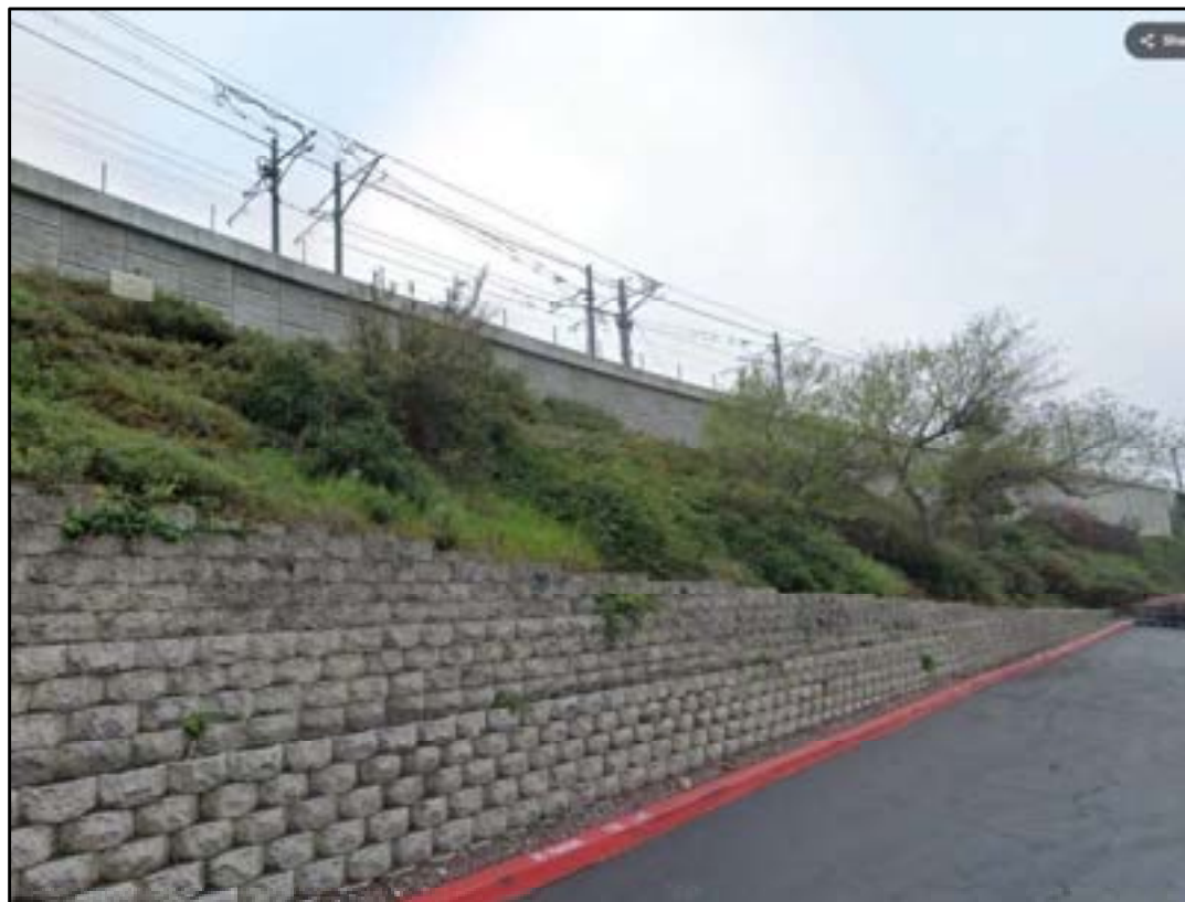
Figure 2-7: Tiered MSE and Keystone Walls along Green Line
