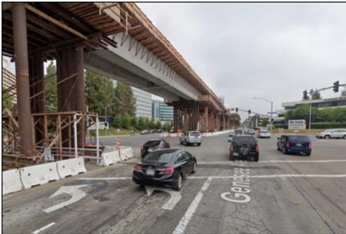
Figure 3-26: Blue Line Construction on Genesee Avenue
