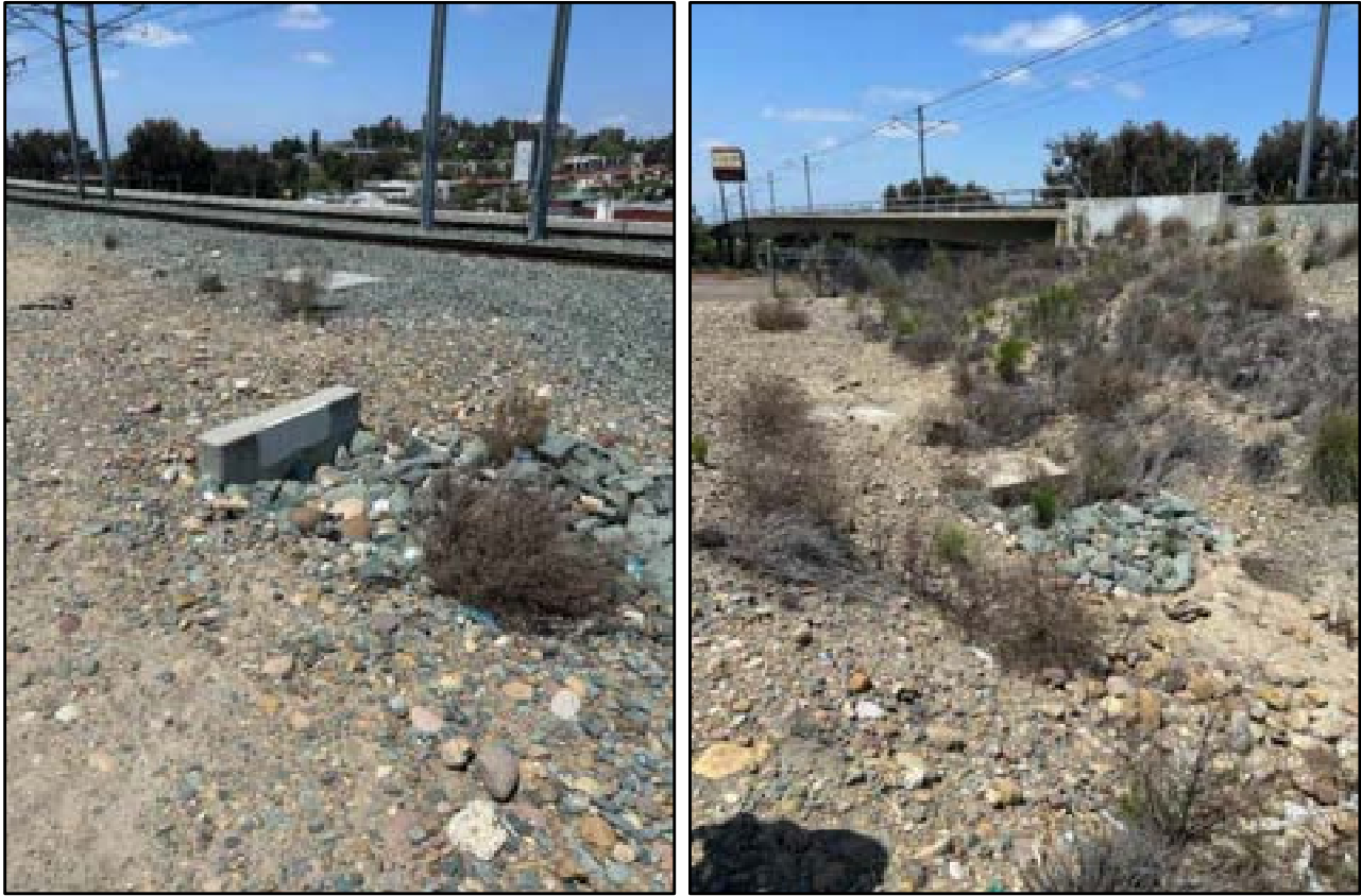
Figure 2-9: Drainage Culvert Headwalls
