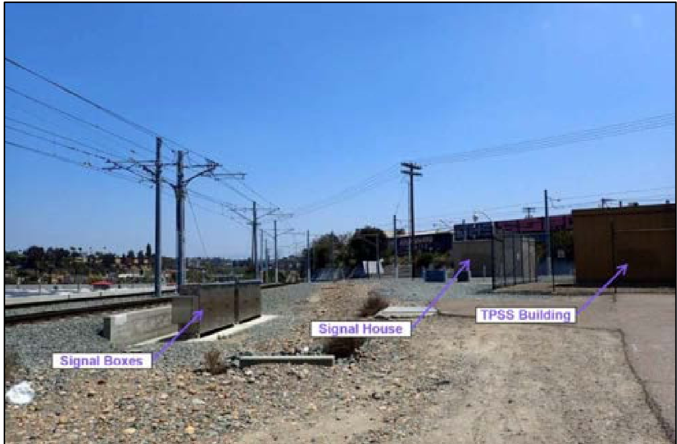
Figure 3-17: Existing TPSS Building and Signaling Infrastructure
