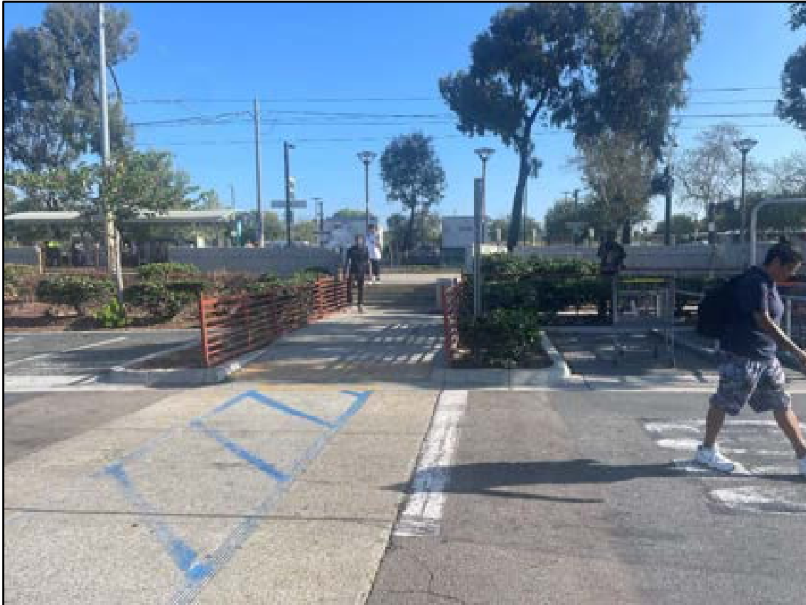
Figure 3-8: Existing South Side Station Access
