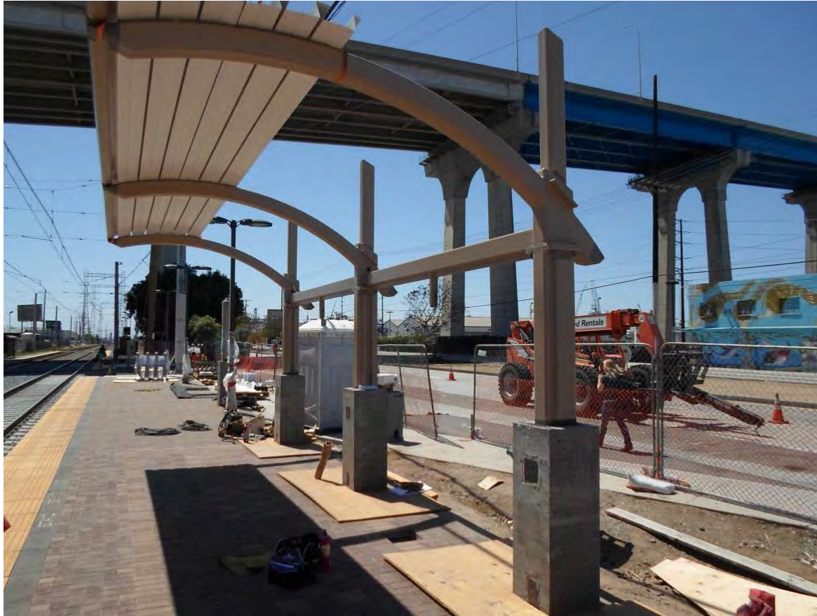
Pavers Installed / Shelter Going In
