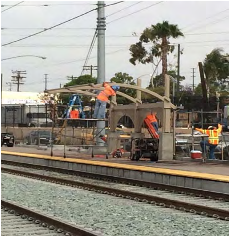
Installing Shelters and Pavers
