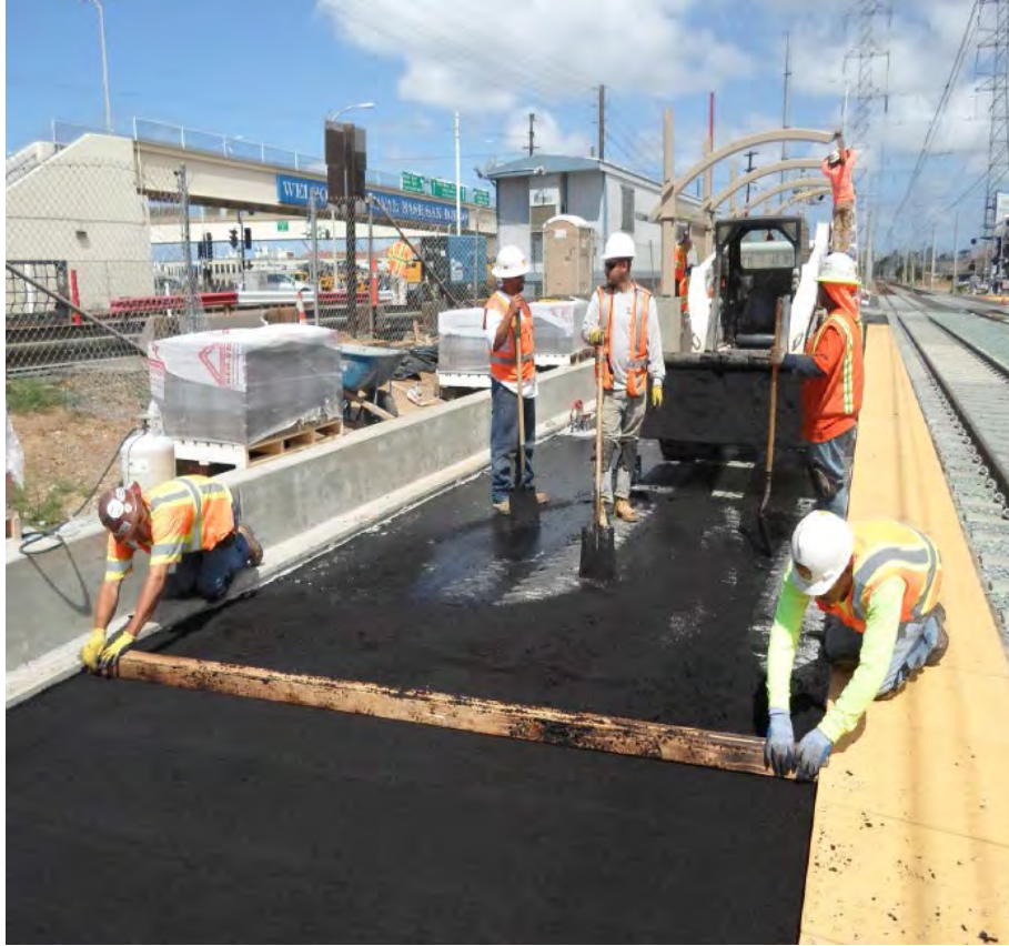
Installing Shelters, Laying Bituminous Bed and Installing Pavers
