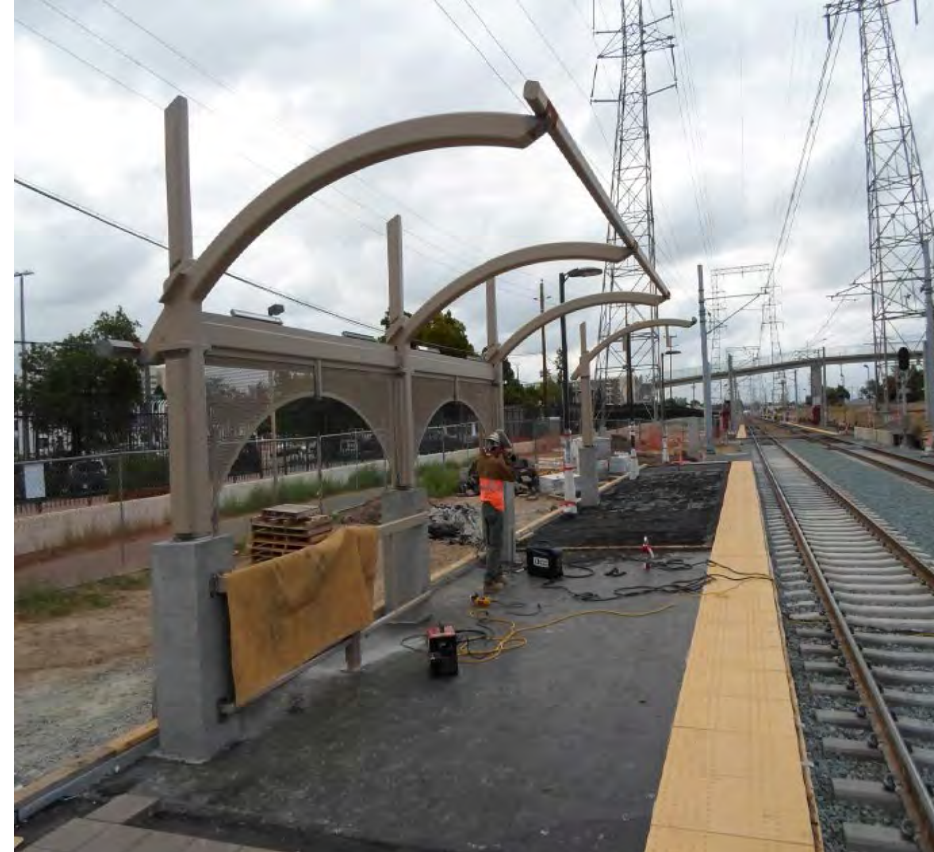
Installing Shelters, Laying Bituminous Bed and Installing Pavers
