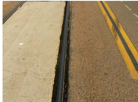
Figure 6-7: Typical Rail Flange Gap
