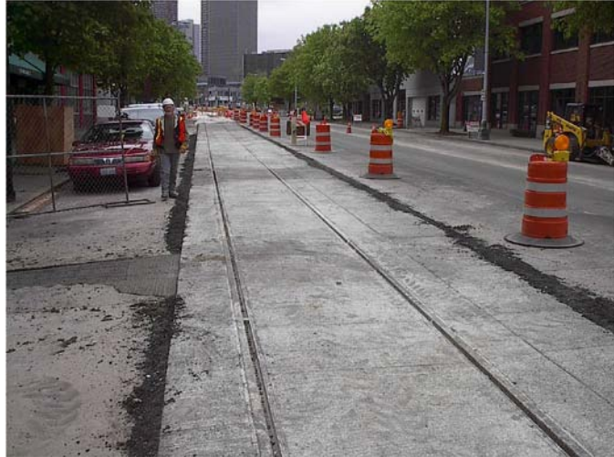
Figure 8-2: Paved Track Nearing Completion in Portland
