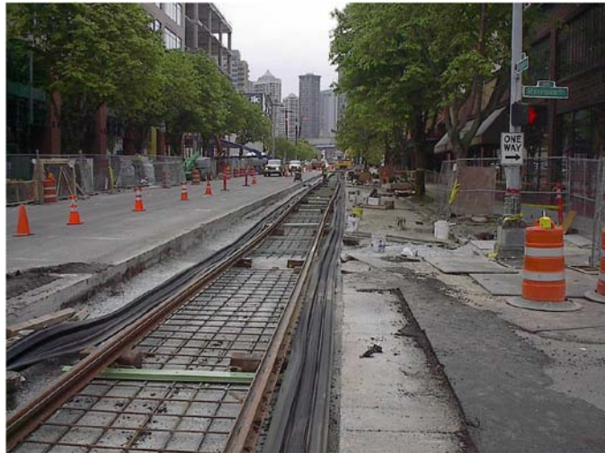
Figure 8-1: Guideway and Track Construction in Portland
