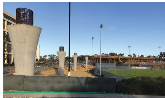
Breaking Ground: Mid-Coast Trolley Extension
