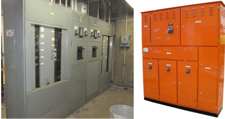
Exhibit 2: Interior switchboard & exterior switchboard
