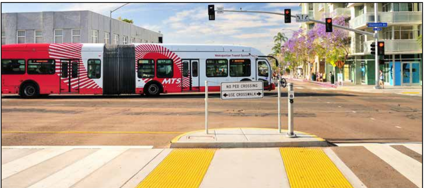
Figure 3-1 Protected Pedestrian Median Refuge
